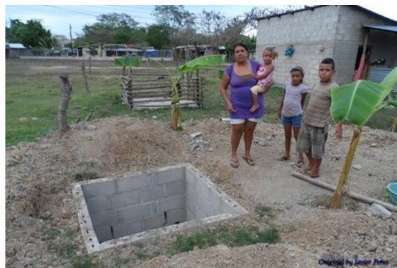
*Family with a partially completed latrine. Next they will get funds for the 'plancha', the concrete top which encloses the latrine and upon which the seat is fastened.*
